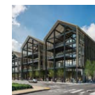
Nashville Warehouse Co. 200,000 SF 20% Preleased AJ Capital Partners UNDER CONSTRUCTION
